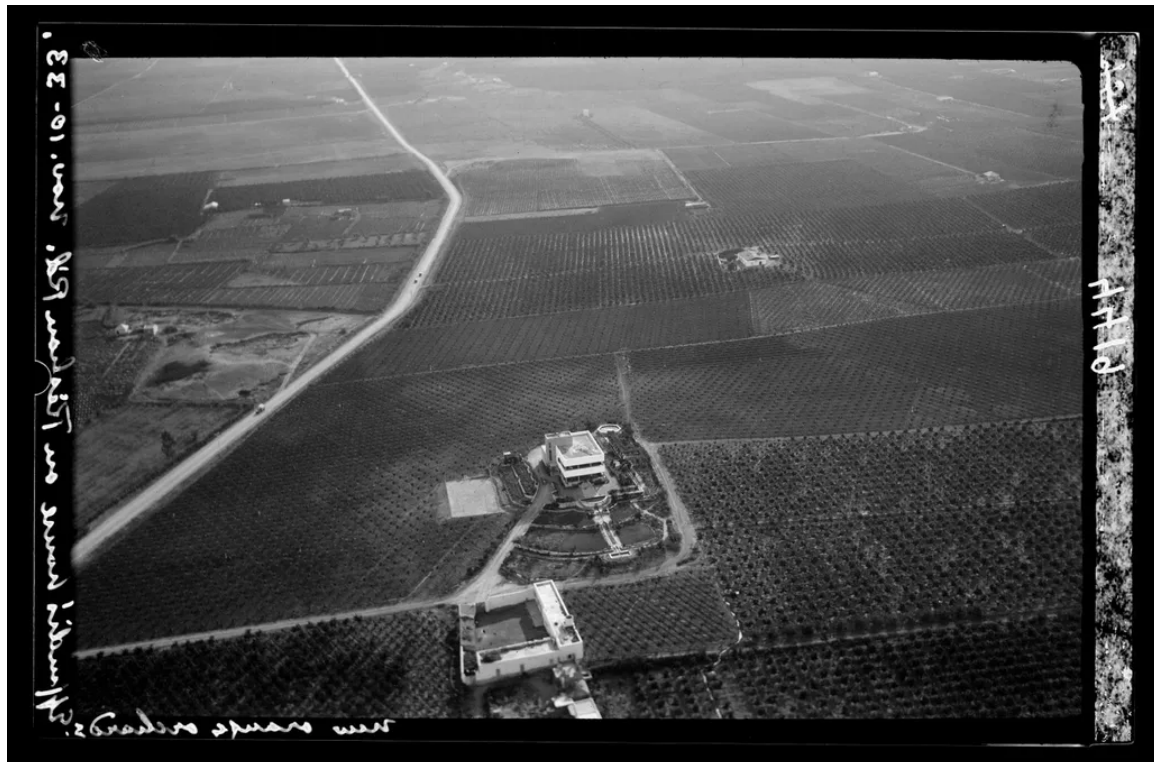
The Abu Aljiban house before demolition, on the outskirts of the village of Beit Dajan. 'All three of them - the landlord, the house and the village - rest in peace,' the tour guide says. Credit: G. Eric and Edith Matson Photograph Collection / Library of Congress
